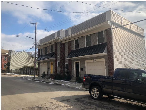
New construction across st from subject property.
