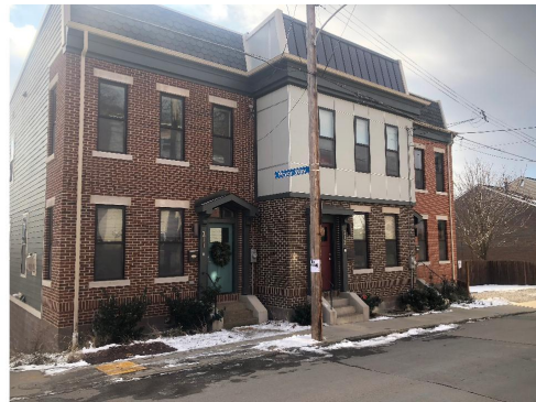
New construction on adjacent st from subject property
